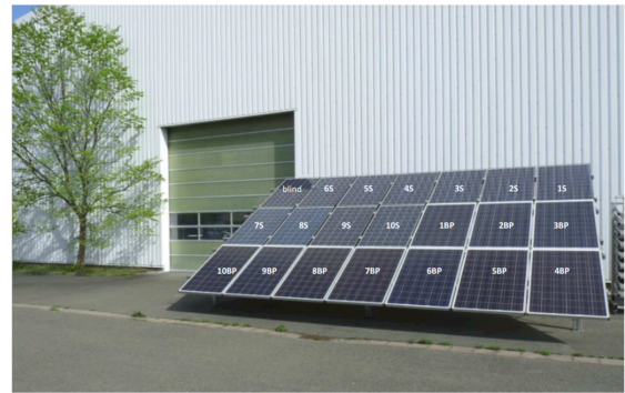
Figure 1: Test-site for Failure simulation on PV-modules in Isseroda, Germany. PV- modules are from Scheuten on the top (1S-10S) and PV-modules from BP Solar (1BP-10BP). All modules are equipped with SunSniffer®-Sensors.
