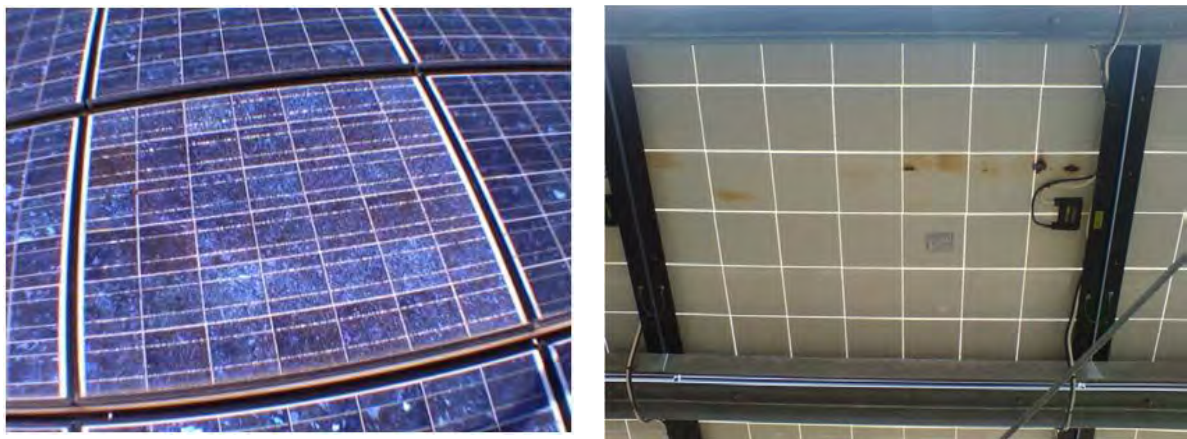
Fig. 6.2.17: Final stage. Left: glass breakage of a PV module caused by broken cell interconnect ribbons. Right: burn marks on the PV module rear side caused by broken cell interconnect ribbons.
