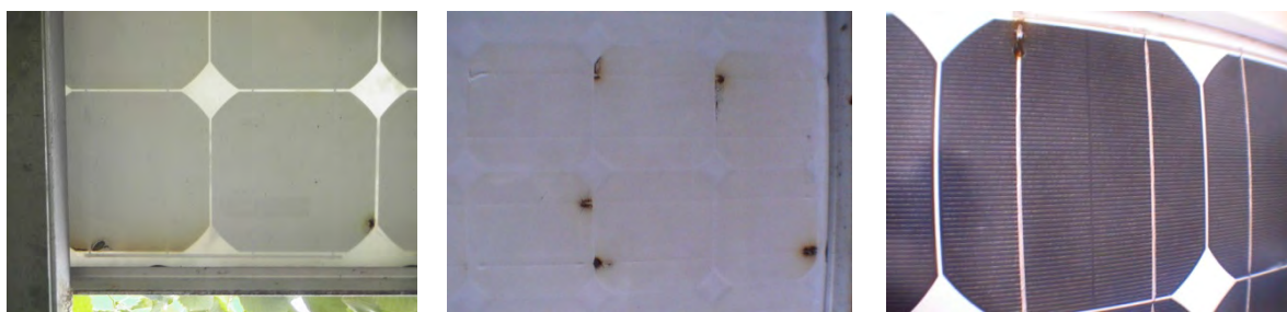
Fig. 6.2.22: Burn marks caused by open-circuit bypass diodes.
