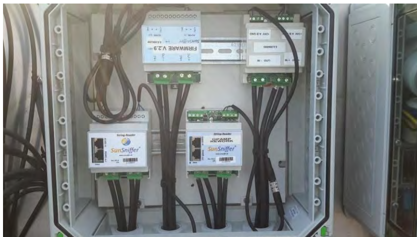
Figure 10: String Readers connected by RS-485 data lines in a water-proof housing.
